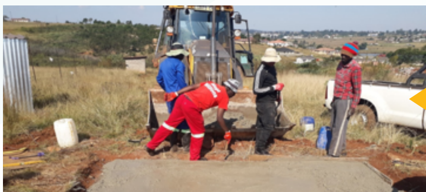
Dumpsite Field Toilet Installation
